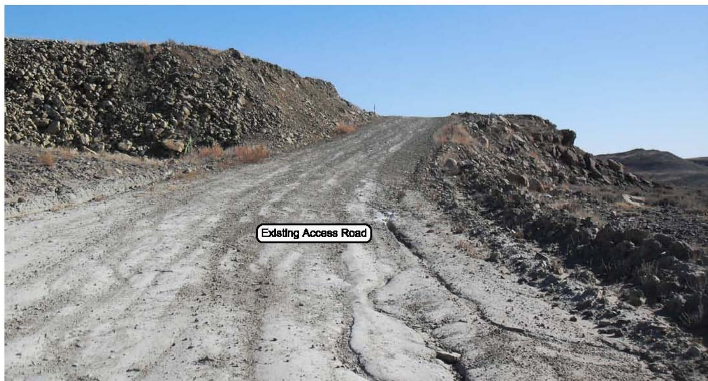
PHOTO VIEW: EXISTING ACCESS ROAD
